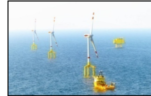
BorWin1 Offshore Light 400 MW
