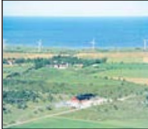
Gotland Light 50 MW IGBT + Plastic cable
