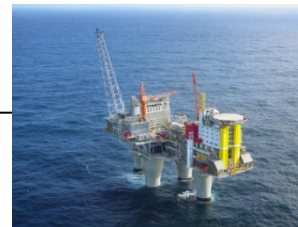
Troll power from shore 84 MW IGBT
