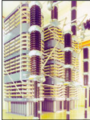
Skagerrak 1-2 500 MW thyristor valves
